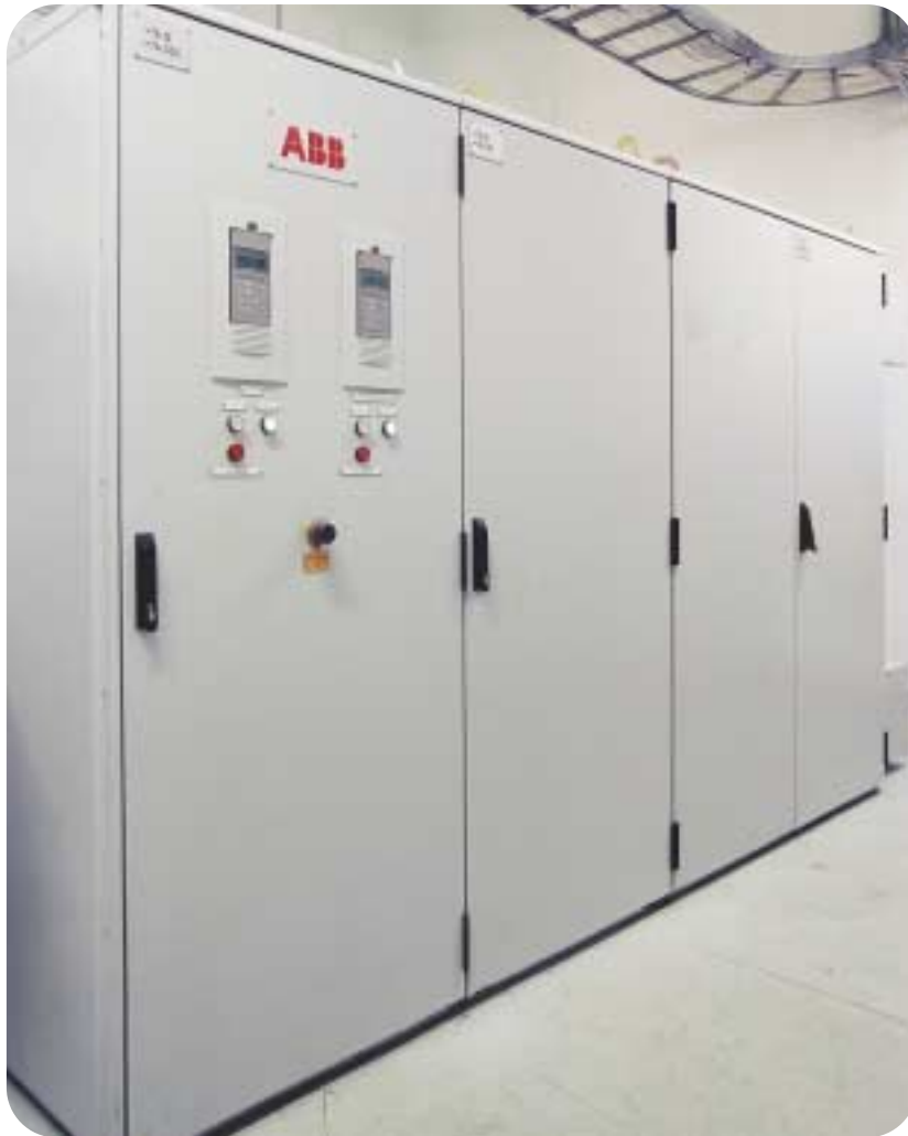
Fig. 5. ACS 6000SD synchronous motor drive.
