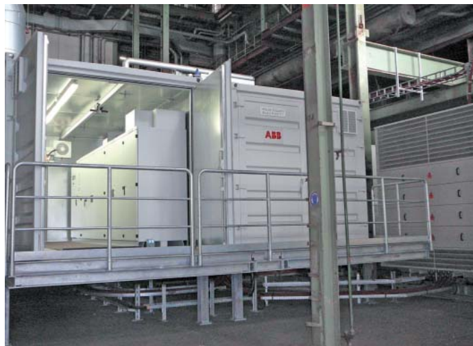
1 GKM power plant, Mannheim, Germany | 2 The water-cooled ACS 1000 medium-voltage AC drives were installed ready for connection in special, fully air-conditioned containers
