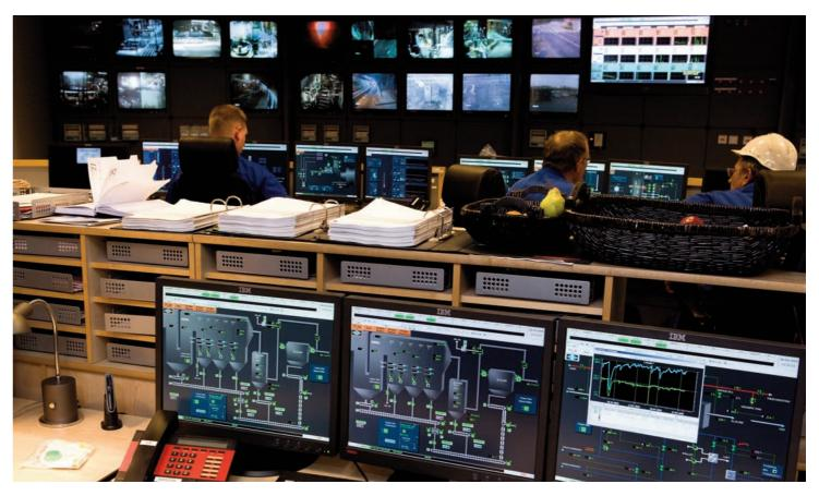
The project scope included design, supply, assembly and commissioning of components and instruments for automation, supervision, control and protection of the entire power station, including critical boiler and filter systems based on System 800xA technology. ABB also supplied Medium Voltage switchgear, SCADA and a protection system.
