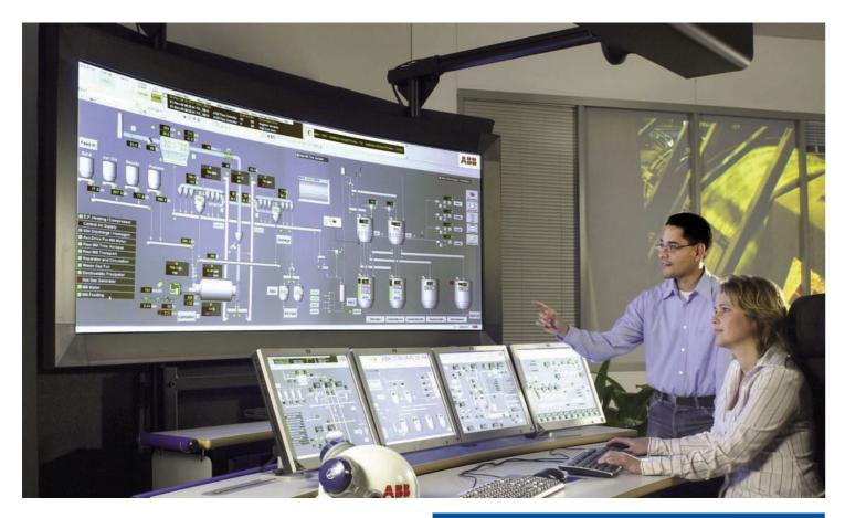
ABB has responded to this demand with its System 800xA, which provides a consistent and intuitive workplace for the management and automation of power generation plant – either within a single site or multiple plants across different locations – using both ABB controllers or third-party systems. It covers both the automation and electrical areas of the plant, so that operators have every device or subsystem under control in a consistent and intuitive environment.
