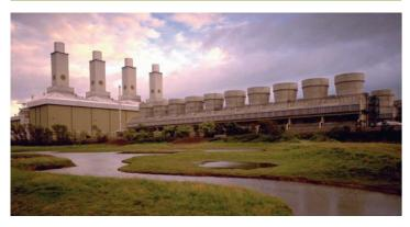
In 2009 ABB completed a major contract from E.ON UK to replace the existing VAX-based operator stations at its 1,420 MW Connah's Quay Combined Cycle Gas Turbine Power Station at Deeside, North Wales with new MS Windows-based power generation portal consoles
