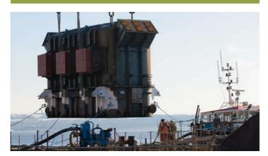
ABB's fast-track transformer re-manufacturing service is currently working on its greatest ever challenge, to repair a failed GSU (generator step-up) transformer at Scottish Power's Longannet power station in Fife, Scotland. At a dry shipping weight of 270 tonnes, the transformer is the largest single unit ever repaired by ABB.
