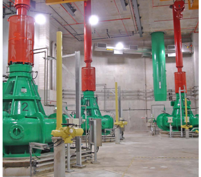
Pumps in one of the two giant pump shafts at the Changi influent pumping station. The pumps are controlled by ABB's ACS 1000 drives.
