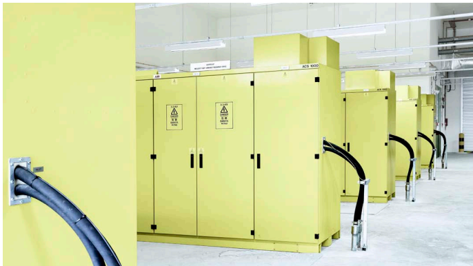
ACS 1000 variable speed drives controlling the pumps.
