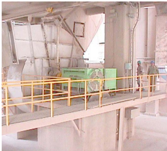
The 10 year old fixed speed fan motor, now controlled by the ACS 1000, operates more efficiently and quieter than before.
