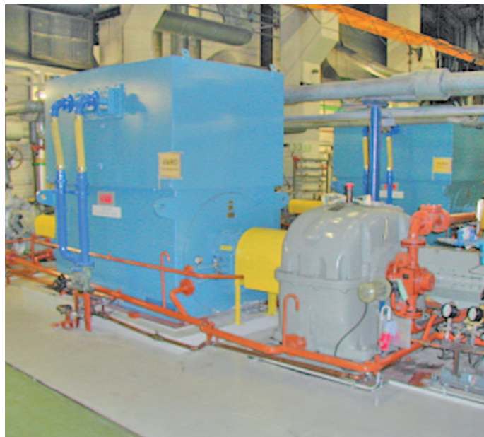
A feedwater pump drive train: the gearbox in front, main pump to the right, booster pump behind the 2-shaft induction motor.
