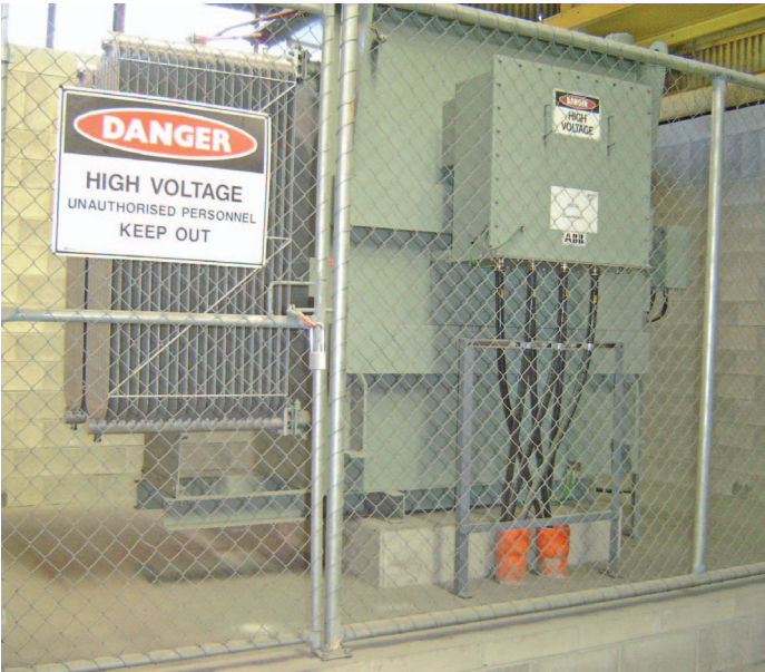
ABB's scope of supply includes high-voltage input transformers rated at 2.8 MVA and UniMix medium voltage switchgear
