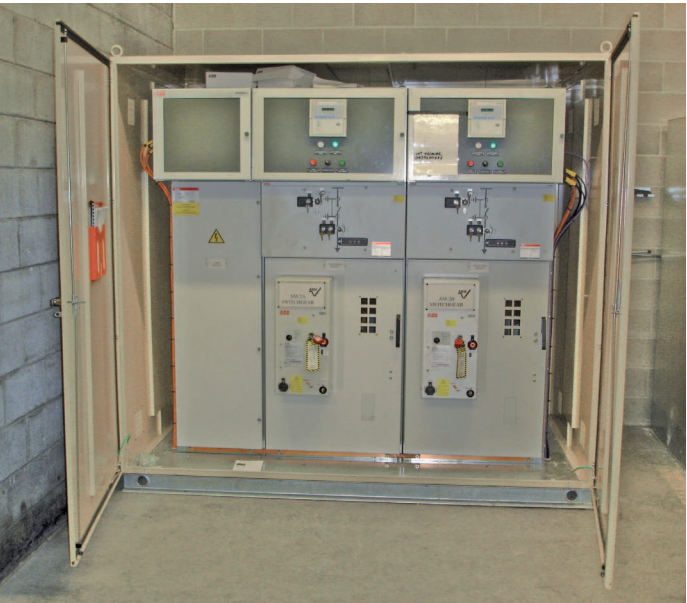
ABB's scope of supply includes high-voltage input transformers rated at 2.8 MVA and UniMix medium voltage switchgear
