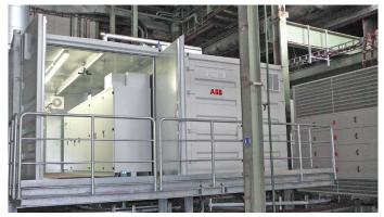
The water-cooled ACS 1000 medium voltage AC drives were installed ready for connection in special, fully air-conditioned containers.
