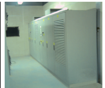
View of the cane mill (862 kW) and ACS 1000 controlling the cane mill at Santa Matilde mill of Compania Azucarera Hondurena S.A..
