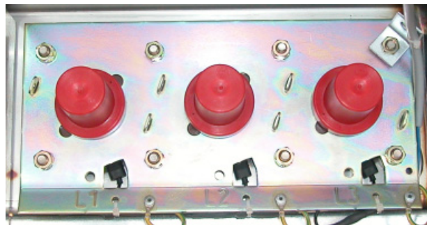
T1 (basic): Plug-in cross member PF250 NF-EN 50181, Connector - Type A (Ir: 250 A, contact finger \varnothing M7.9 ^{+0.02}_{-0.05} mm)
