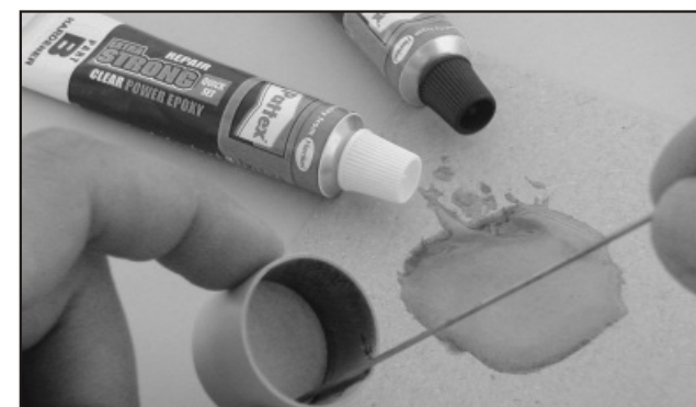
12. Same way to glue another disc in the body of Optical Sight and flushed with cap edge on one end.
