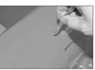
87. Install the engine cowling; first glue the plywood doublers inside the fuselage at where hole is . Trial fit the cowling in place and temporarily secure it with mask tape. Drill 1/16"(1.5mm) at the place where doublers are.
