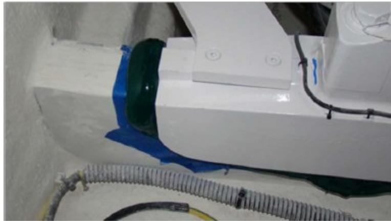
FIGURE 13 – ADHESIVE SQUEEZE OUT
