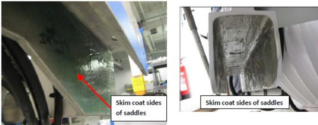
FIGURE 11 – APPLYING ADHESIVE TO SADDLES
