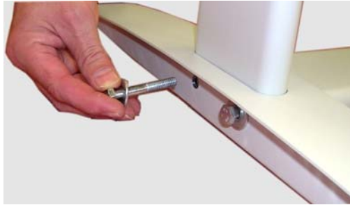
Picture 8: Inserting screws with washer
