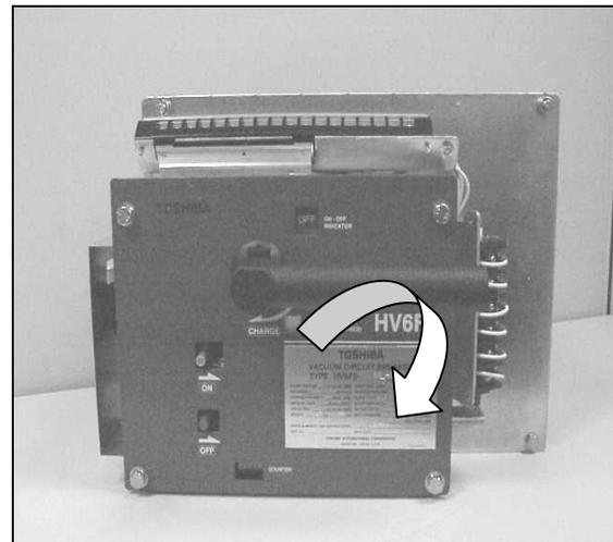
Fig. 23 Preparing to Manually Charge Breaker
