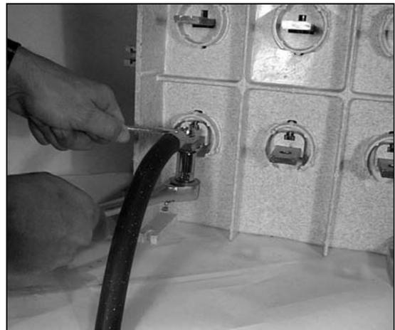
**Fig. 16 Fasten Cable to Main Circuit Terminal**
