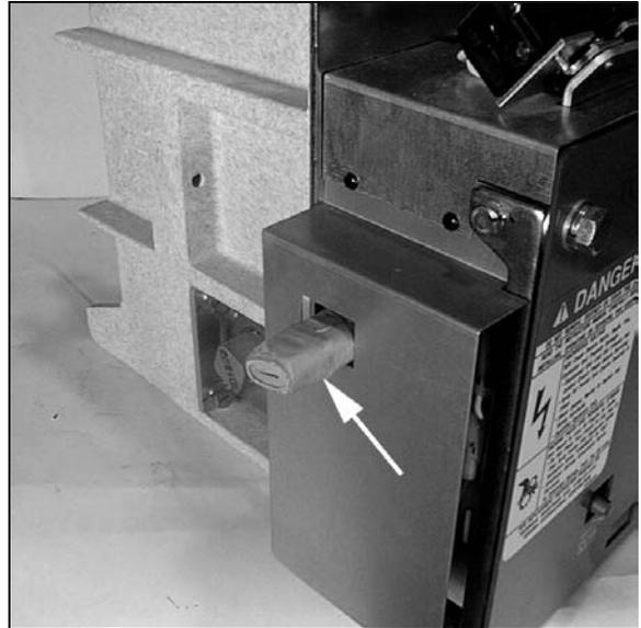
**Fig. 30 Plug Installed in UV Trip Device**
