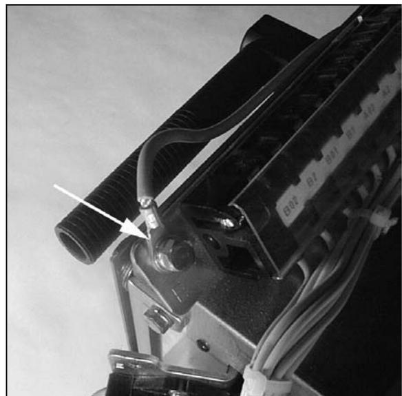
**Fig. 19 Ground Connection for ML Type Breakers**
