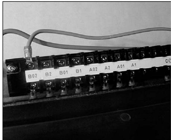
**Fig. 22 Auxiliary Contact Connections on ML Type Breakers**
