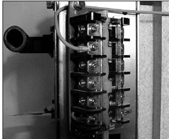
**Fig. 21 Auxiliary Contact Connections on MU Type Breakers**
