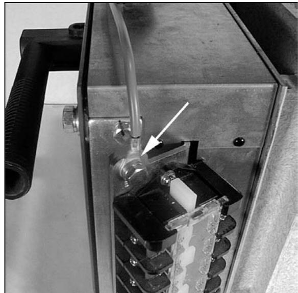
**Fig. 18 Ground Connection for MU Type Breaker**
