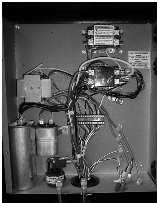
Figure 13. AE-Ti Control Panel, Interior View
