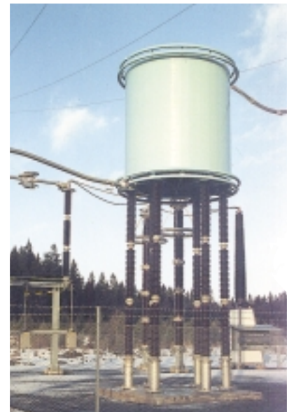
Fig. 17 HVDC-Smoothing reactor
