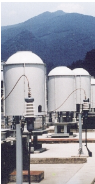
Fig. 35 Filter reactor with sound shield
