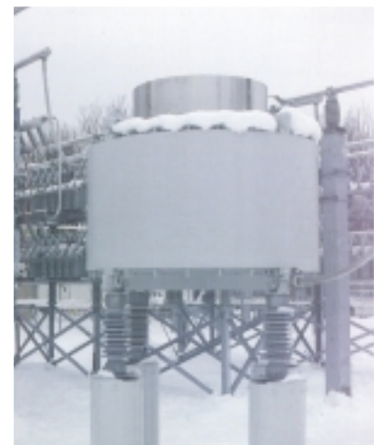
Fig. 9 Filter reactors with de Q'ing rings
