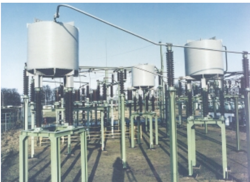
Fig. 3 Single phase series reactors
