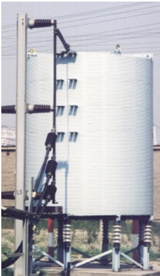
Fig. 5 Buffer reactor for E.A.F.
