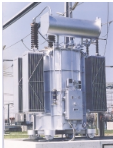
Fig. 27 Arc suppression coil 110 kV
