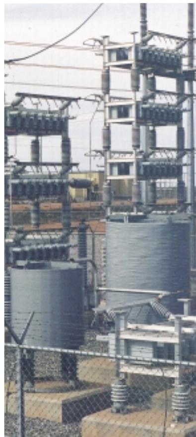
Fig. 8 Filter reactors
