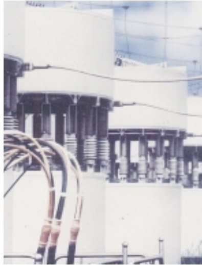
Fig. 12 Tertiary connected shunt reactors
