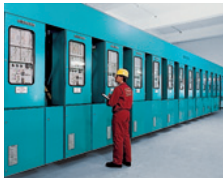
Bay with integrated local control cubicle
