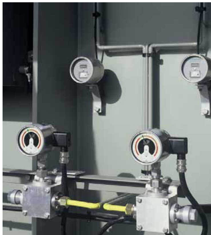
Gas and electrical monitoring for GIS arrester
