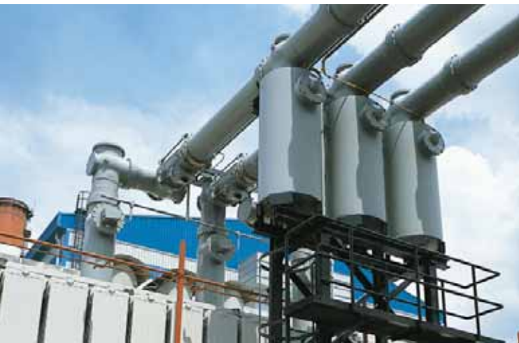
GIS arresters connected to a 420 kV GIS busbar
