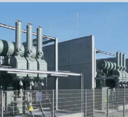
GIS arresters installed at a 123 kV transformer with Oil-SF 6 -bushing
