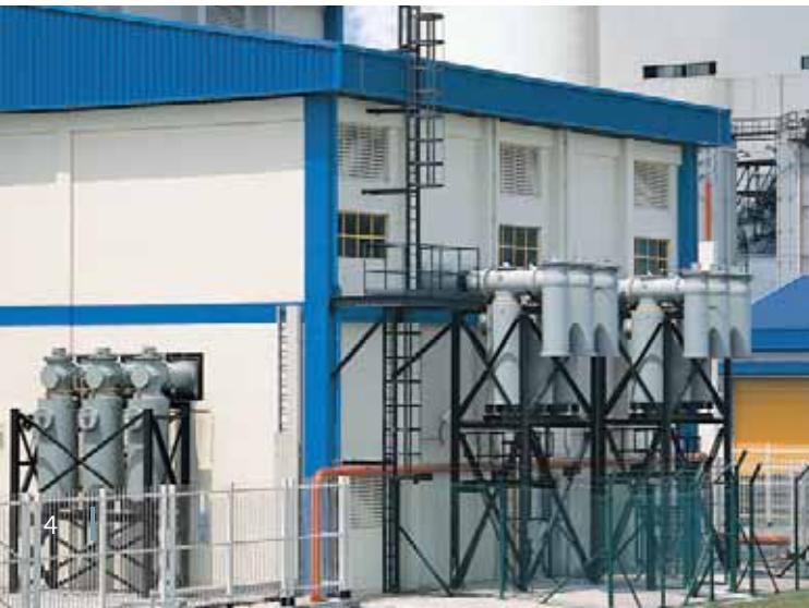
GIS arresters connected to a 420 kV GIS busbar
