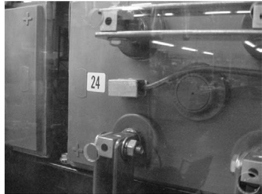
Figure 3.4-3 Battery Probe Installation
