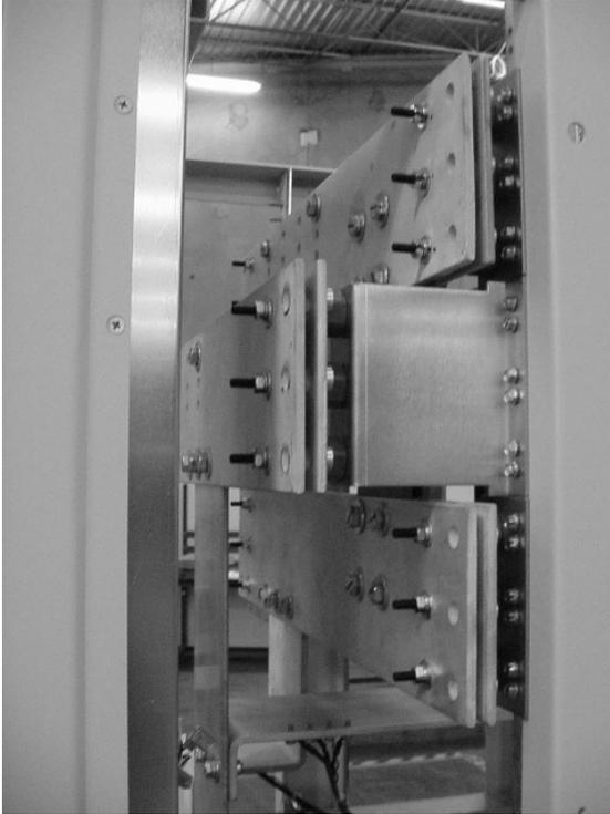
**Figure 3.2-2 MX28B-1200-2400 has a maximum capacity of 2400 Amps.**
