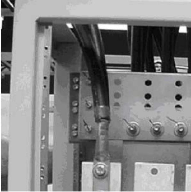
Figure 3.5-1 DC System Grounding
