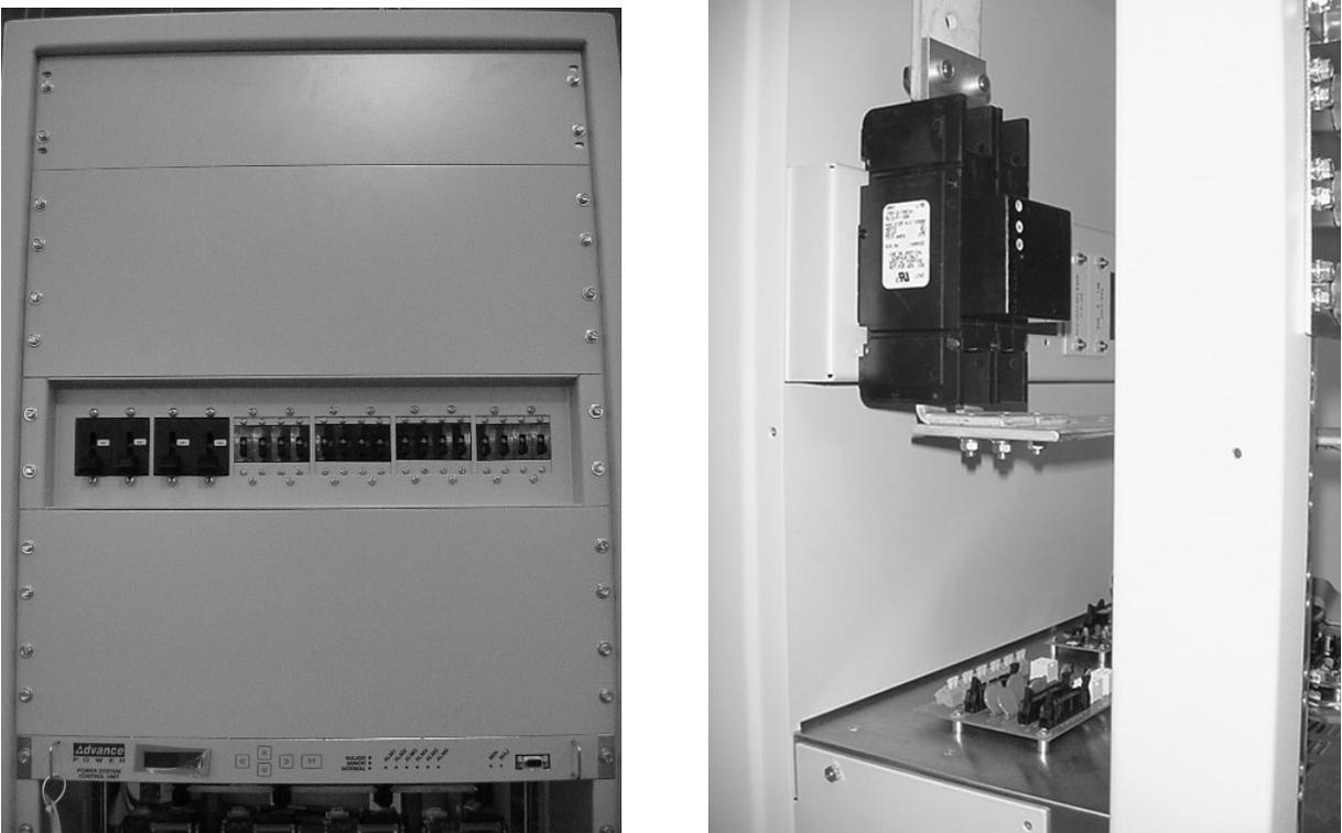
Figure 3.6-4 Bolt-in Circuit Breakers
