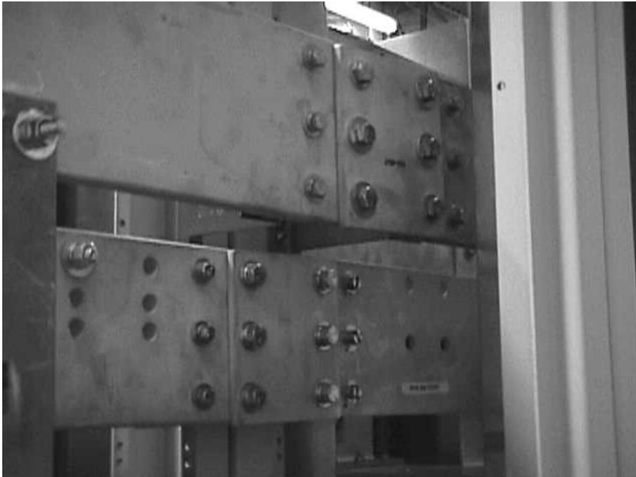
**Figure 3.2-4 Splice Plate Installation**
