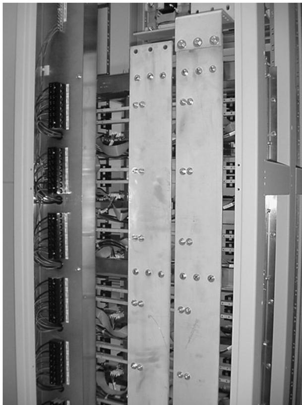
**Figure 3.3-1 AC Input Wiring**
