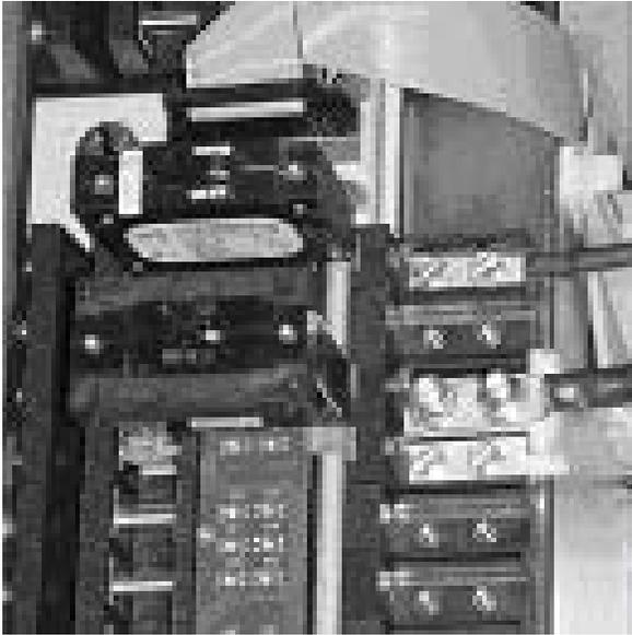
**Figure 3.8-1 Load connections for snap-in breakers**
