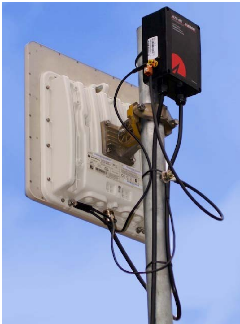
Figure 79 - Upper Grounding Configuration
