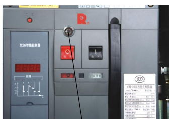
“分闸”锁定装置 “Break” lock mechanism
