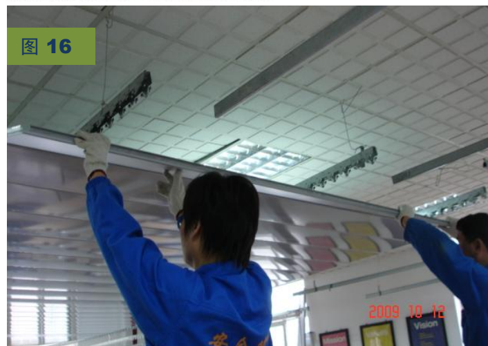
图 16 Two people install or remove the panels 需两人安装或拆卸面板
