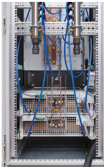
带水冷装置的混合机柜系统 / Mixed system with water cooling
