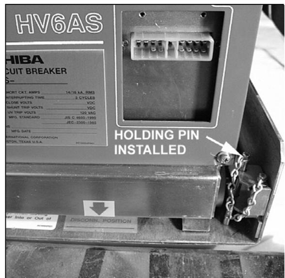
Fig. 20 Breaker at DISCONNECTED Position
