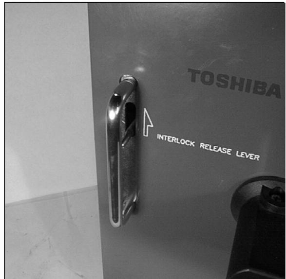
Fig. 3 Interlock Release Lever
