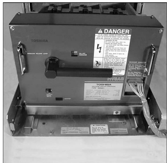
Fig. 22 Breaker at CONNECTED Position
