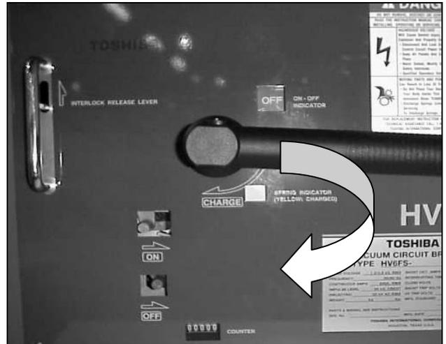
Fig. 25 Preparing to Manually Close Breaker
