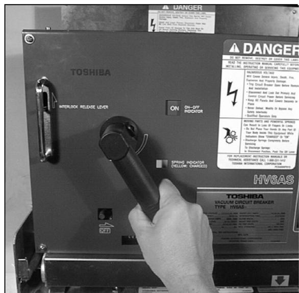
Fig. 26 Manually Charging Breaker
