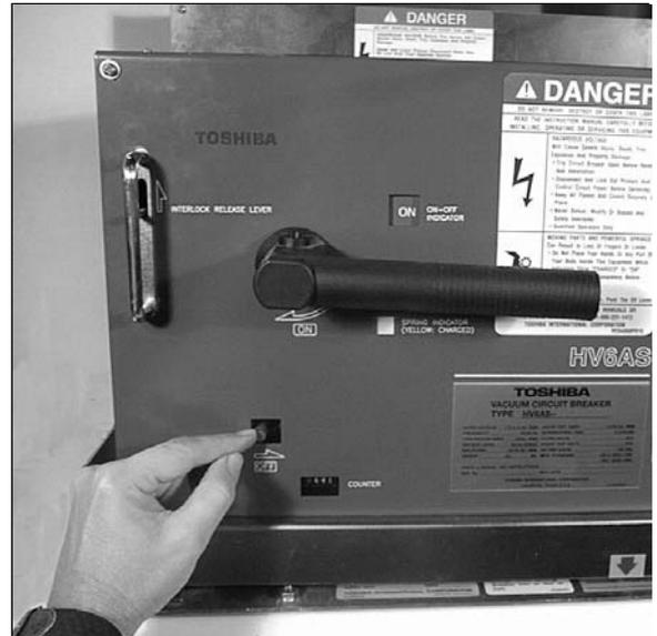
Fig. 27 Manually Opening Breaker
