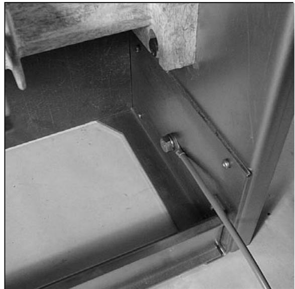
Fig. 14 Installation of Ground Wire
