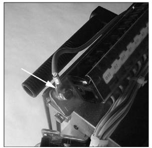
Fig. 19 Ground Connection for ML Type Breakers
