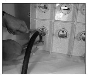
Fig. 16 Fasten Cable to Main Circuit Terminal
