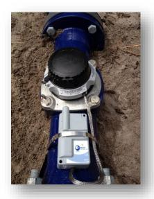
WASP-2G-1FL secured with stainless steel cable tie
