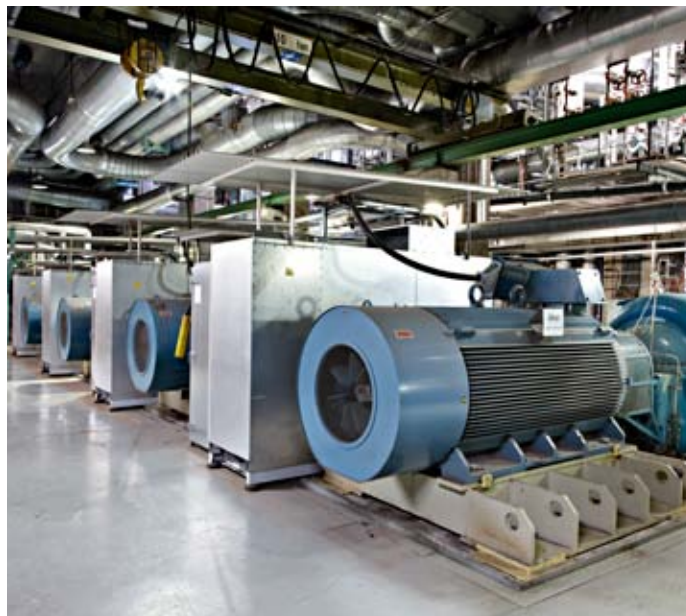
View of the ACS 1000 drives, motors and district heating pumps at Mälarenergi's power and district heating plant in Västerås
