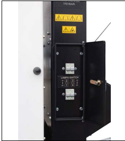
Figure 6.4 – Light control switches
