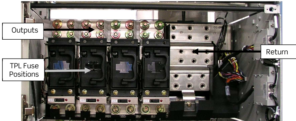
Figure 24 - TPL Fuse Panel
