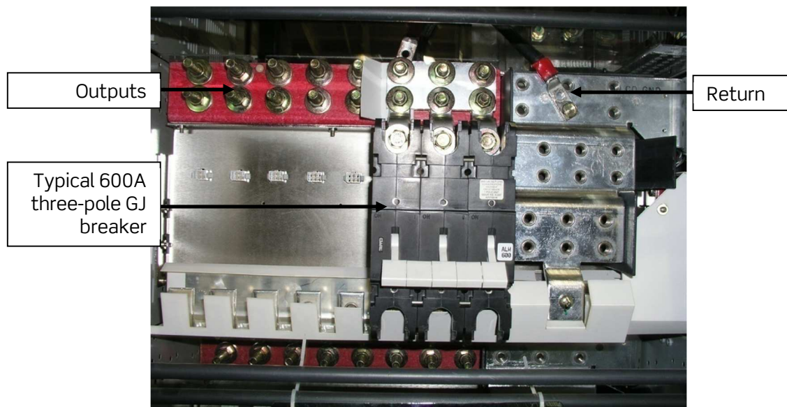
Figure 23 - GJ / GS Breaker Panel (with breaker installed)
