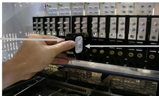
Figure 22 - DC bullet breaker panel
