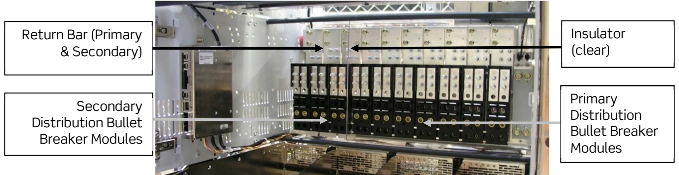
Figure 4 - MDP Panel with BG2 Modules Installed
