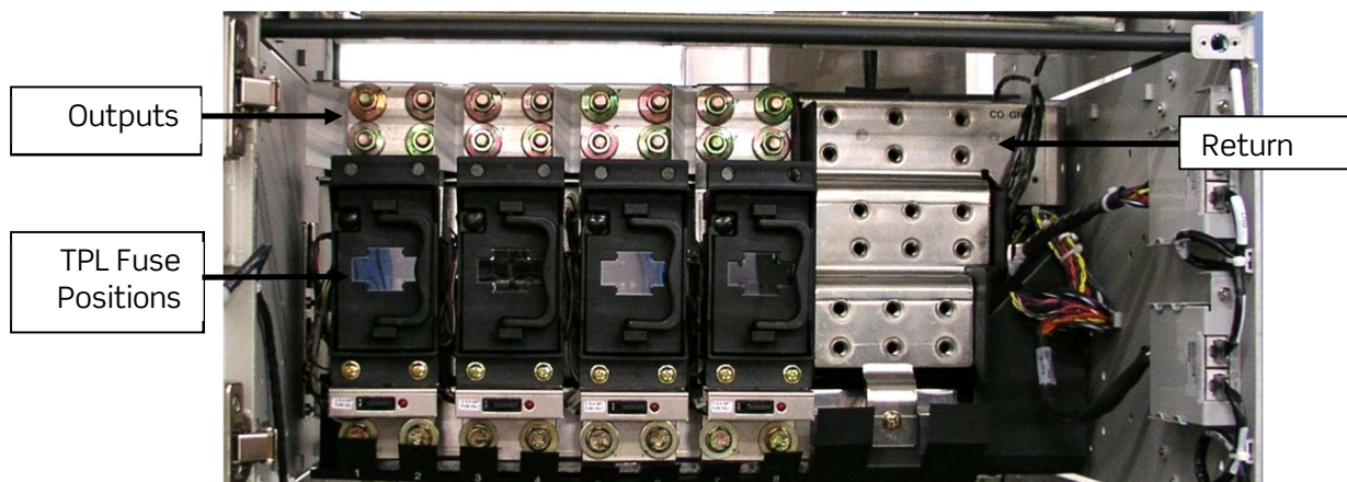
Figure 6 - MDG Panel with TPL Configuration
