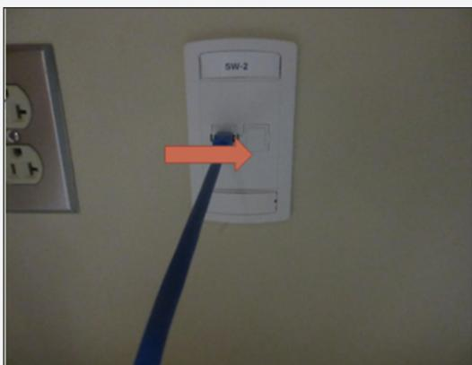
**Figure 40 :** Check that the network cable is plugged securely into the correct jack.
