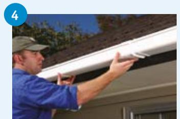
Solvent cement replacement section into damaged area. Remove any excess Marley solvent cement (MCS®).
