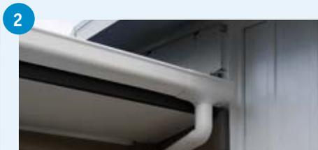
Re-insert spouting into expansion outlet. Ensure end of spouting aligns with temperature marking on inside face of outlet.
