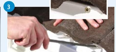
Secure spouting to fascia using a screw at the point furthest from the expansion outlet in the same run. This will control movement to and from the expansion outlet.
