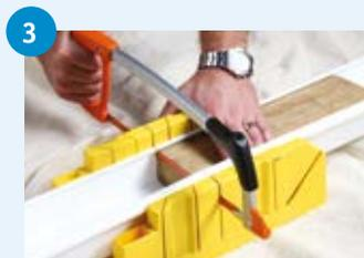
Cut replacement section on ground and solvent cement a joiner and expansion joiner to each end.
