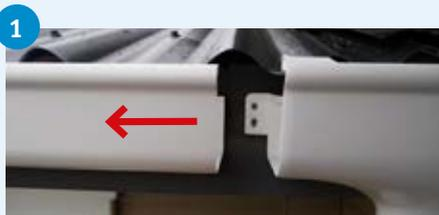
Spouting creep is when expansion and contraction does not occur in a conventional manner and may result in spouting pulling out of the expansion outlet or pushing into outlet and causing blockages.
