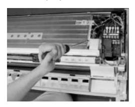
10) Remove the Thermistor of the Evaporator.
