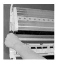
18) Remove 4 screws fixing the Side cover R, and pull the Cross flow fan
