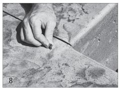
Insert plastic anchors (33) into the holes and tap with a hammer so they are flush with the deck. Fasten the lid to the deck with #12 pan head screws (26).
