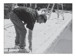
Pull the rope down the back side of the guide toward the cover housing.
