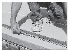
Hold the rope outside the guide to pull the rope down the length of the guide toward the end of the pool.
