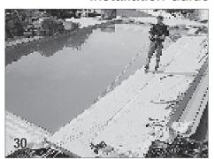
**Attaching The Ropes To The Reels**Pull the cover back until the sliders are against the stops. Pull the ropes tight as they come off the pulleys on the mechanism to eliminate the slack in the rope.
