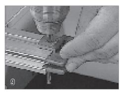
Holding the guide feed firmly, use a 6 inch 3/16"bit to drill through the hole in the guide feed and through the guide. Remove the guide feed. Do this for the guide on both sides of the pool.
