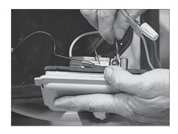
Insert the hot wire from the power supply into terminal L1 on the back of the switch and tighten the screw.
