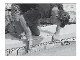
Insert and tap the spacer into place underneath the guide along the entire length of the guide. Do this along both sides of the pool. The spacer needs to end at the inside edge of the housing
