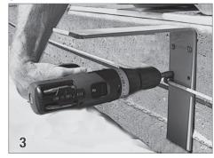
Secure the brackets to the back wall of the housing using #12 x 1½ "hex head screws( 34). Mount a rope loop (30) on one screw of each of the brackets. This will keep the rope running straight along the back of the housing.
