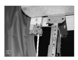
Run #8 copper bond wire (38) from the lug on each guide feed to the lugs on each mechanism end.
