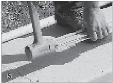
Lay the sections of guide on the deck and tap them together using a rubber mallet so the center splice and splice pins interlock with each section of guide. It's important that, the splice is tight together so there is not a gap from one guide to the next. Slide pulley end cap (15) into the end of the guide at that is at the opposite end of the pool from the mechanism..
