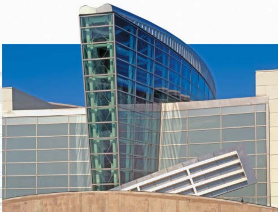
Houston Intercontinental Airport, International Arrivals Terminal Solarscreen™ VE1-2M Silk-screen Houston, Texas Architect: PGAL Wes Thompson Photography
