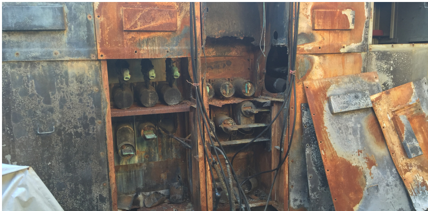
Continuous, real-time monitoring of MV common failure modes (excessive temperature, partial discharge (PD), and humidity) could have prevented the damage inflicted upon this MV switchgear.
