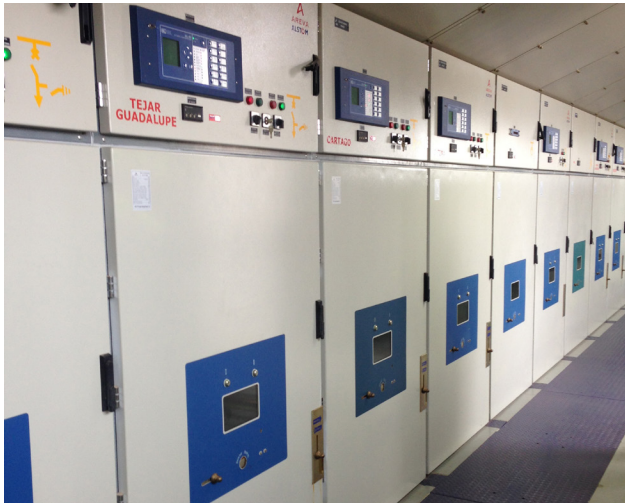
Medium-voltage substation switchgear lineup benefiting from real-time, continuous condition-based monitoring
