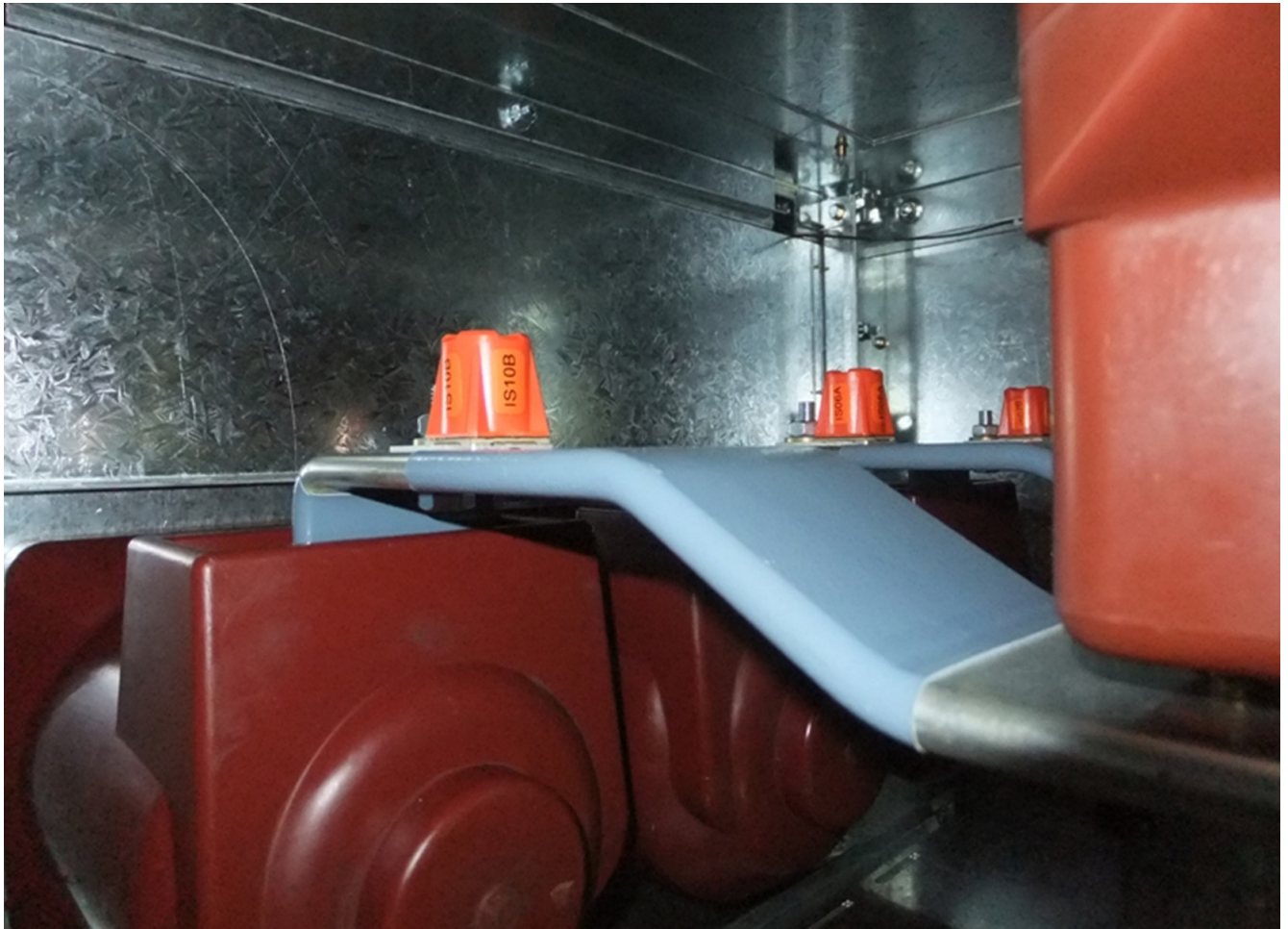
SAW temperature sensors (orange sensors) installed within a MV switchgear at the circuit breaker input and output bus connections
