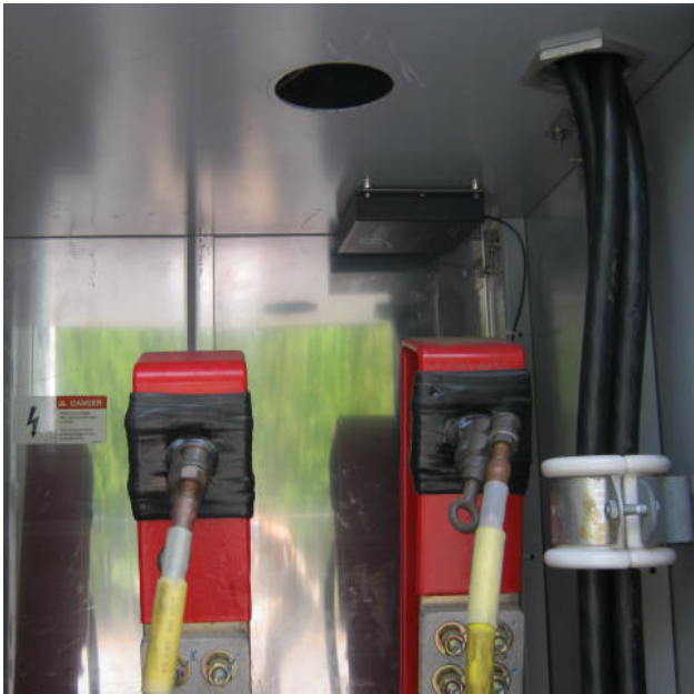
A band-pass UHF partial discharge antenna easily installed in a safe position (upper corner) of a MV bus tie
