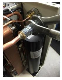
Figure 16 Connect Self-Sealing Coupling
