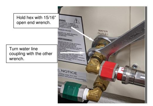
Figure 5 Connect and Remove the Water Lines
