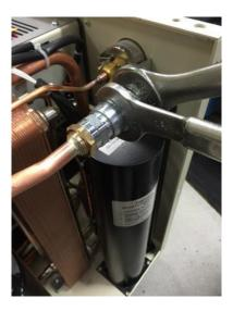
Figure 9 Disconnect Self-Sealing Coupling
