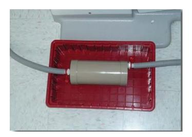
The Chairside amalgam separator will need to be changed when vacuum levels fall below recommended values (see the manual for additional details). The used amalgam separator (still connected to the vacuum lines) should be placed in a tray that will collect any spilled wastewater, preventing it from contacting the Operating floor.
