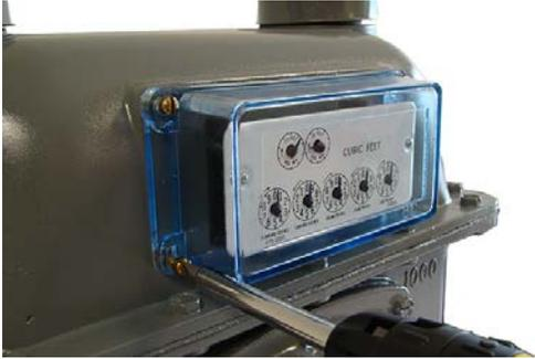
2. Remove the two index screws in an alternating fashion. Loosen the left index screw two turns, loosen the index screw three to four turns. Hold the index while removing the screws to keep the index from falling. Set the index aside where it will not be damaged.
