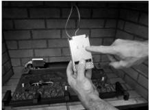
4. Remove the 3 screws holding the bulb assembly in the accent light enclosure. Remove the bulb assembly from the enclosure.
