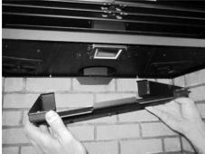
Remove the accent light cover plate from the roof of the firebox. Remove the outer 8 screws, not the inner 4 screws.
