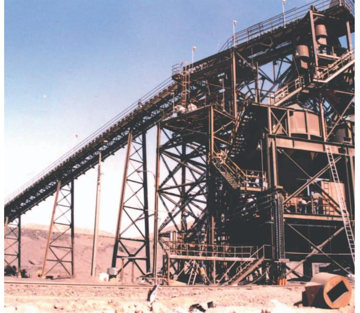
View of the conveyor driven by an ACS 1000 retrofitted to an existing induction motor of 400 kW located on a platform at the top end of the conveyor.
